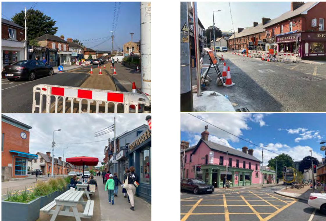
Figure 15 Images showing the road-space reallocation underway in Dundrum Main Street (September 2020 - top), and the works when completed, bottom (images by S. Rock)
