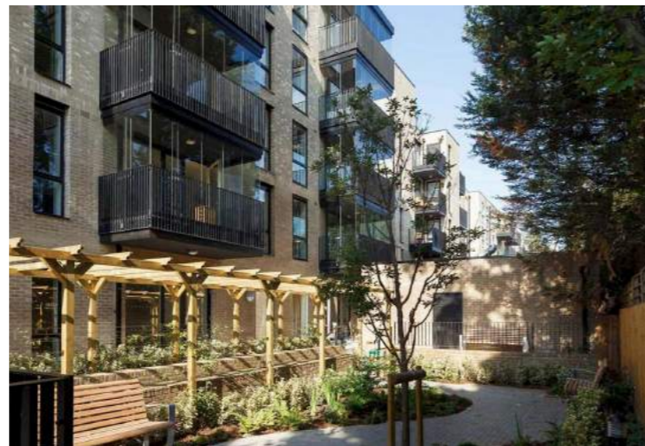
Courtyards provide external space for the older residents
