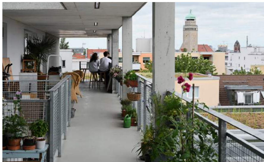
EM2N - HOUSING ON BRIESESTRASSE, BERLIN Allowing more sunlight to enter deck by cutting through slab, added privacy for units with windows facing deck with railings and planting
