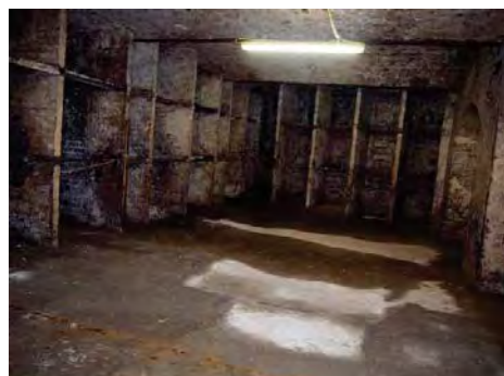
Discovered basement cellars at No. 8-9 Moore Lane
