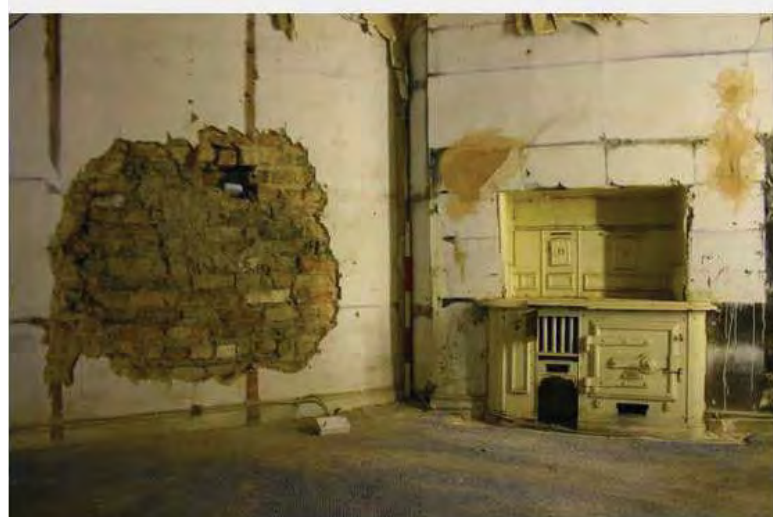
Existing Condition No.17
