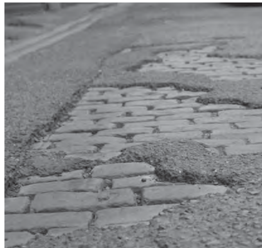
Moore Lane cobble stones surfacing underneath modern tarmac
