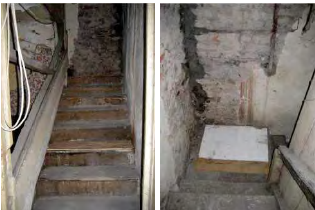
No.14 Re-instated staircase
