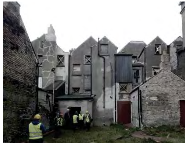
View from the yard towards the monuments
