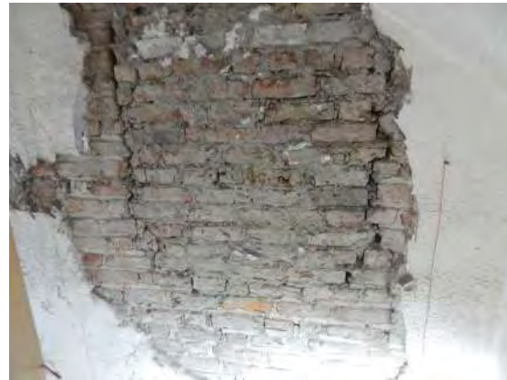
Hole in the wall - refilled no.16
