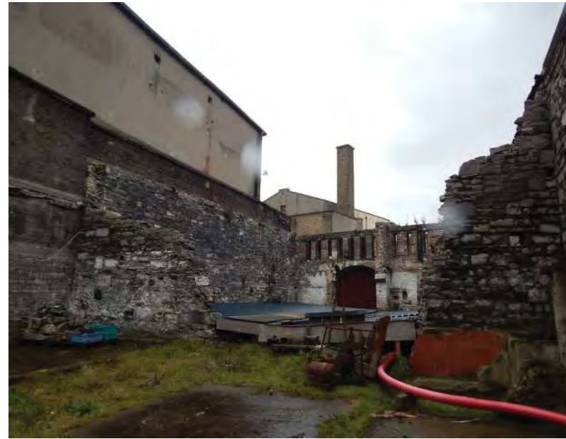
03. Looking towards Moore Lane, remaining stone walls
