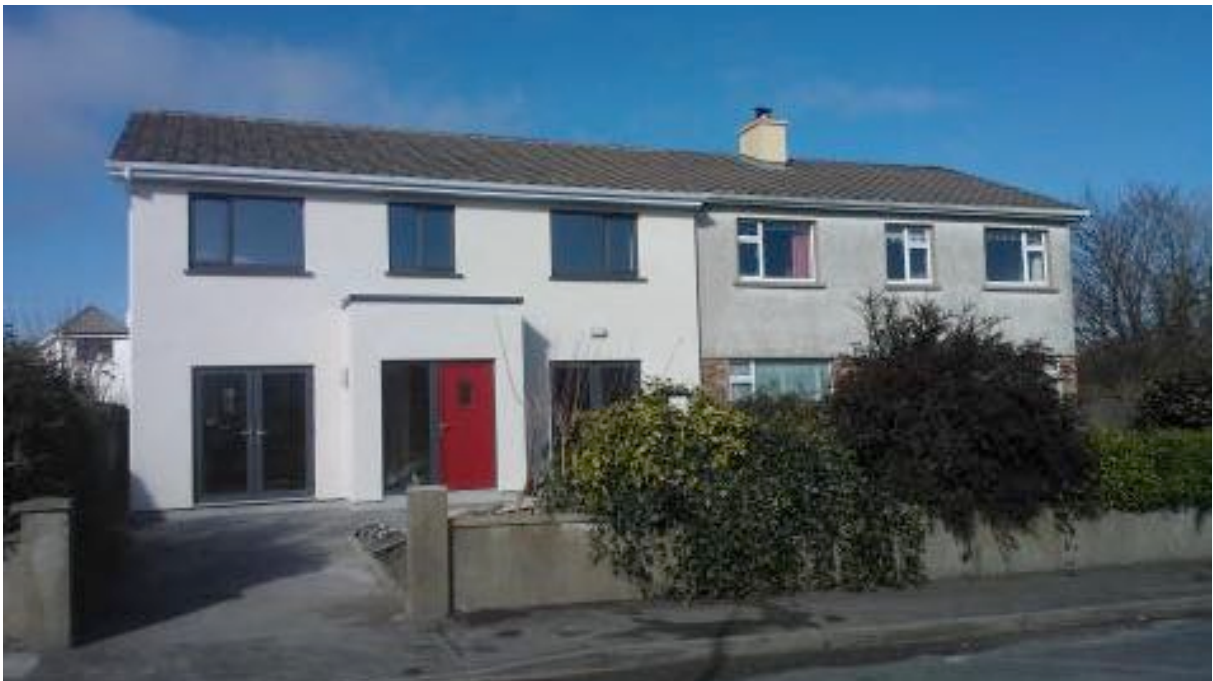
Fig. 5.4 Case-study building - existing dwelling after retrofitting works - view from street.
