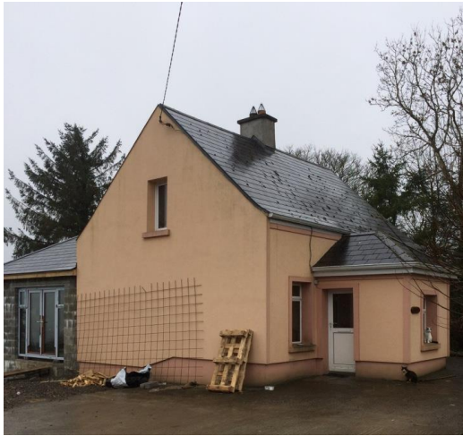
Fig 4.5 Externally insulated home
