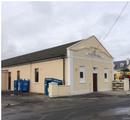
Fig 4.13 Bangor Erris Parish Hall
