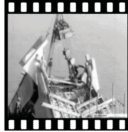
Ridge beam is concrete jointed and tied across with cables.
