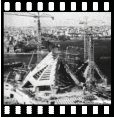
Construction of arch crowns.
