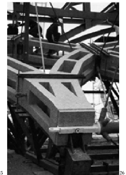
Granite being prepared to hoist
