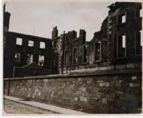
— T.J. Westropp, view of facade from Lisburn Street, 1916.
