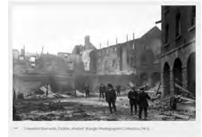
What was left from the fire from 1916
