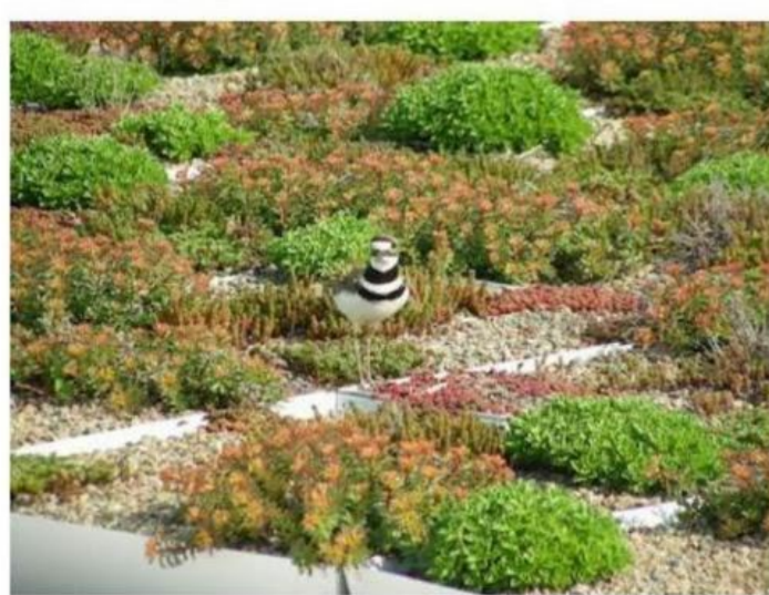
Green Roof Wildlife Habitat
