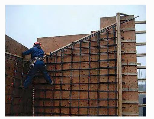
Steel rebar installation between the formwork for the concrete walls.
